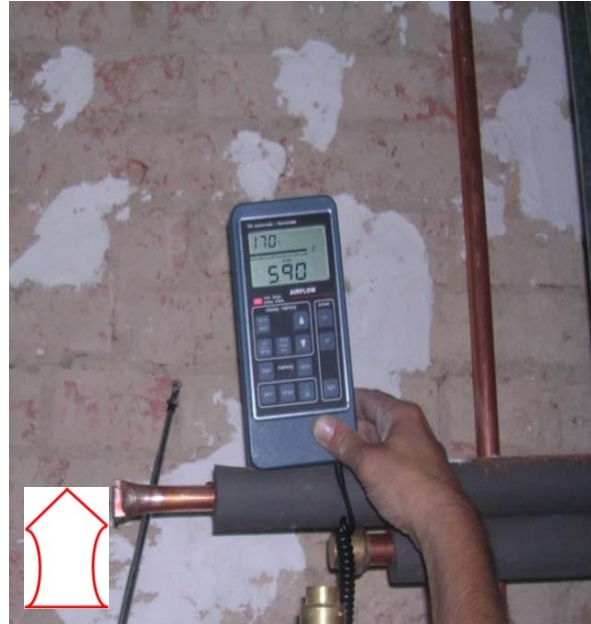
Monitoring during construction process: BlowerDoor test at depressurization
