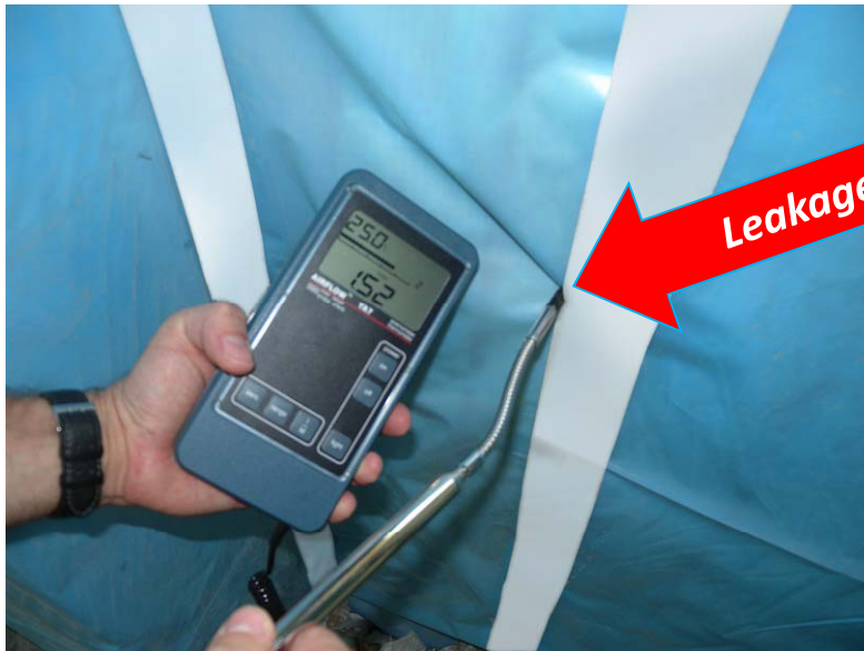
Leakage detection with thermal anemometer
