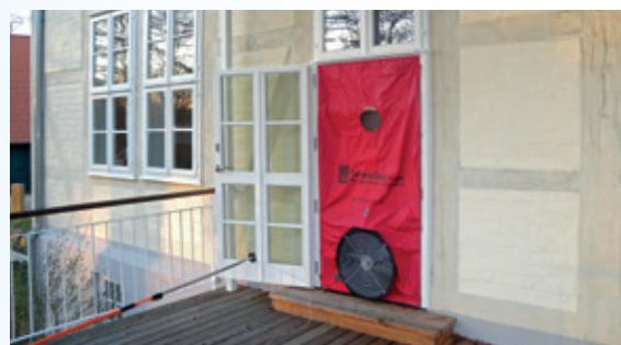
BlowerDoor measurement in the context of an energetic renovation
