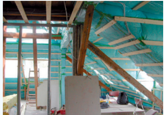
The air barrier is still visible (sheets and wood panels): This is the optimum time for a BlowerDoor measurement.
