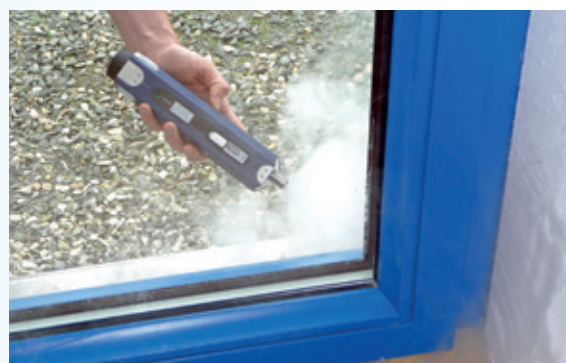
Leakage detection with the fog generator BlowerDoor HandFogger
